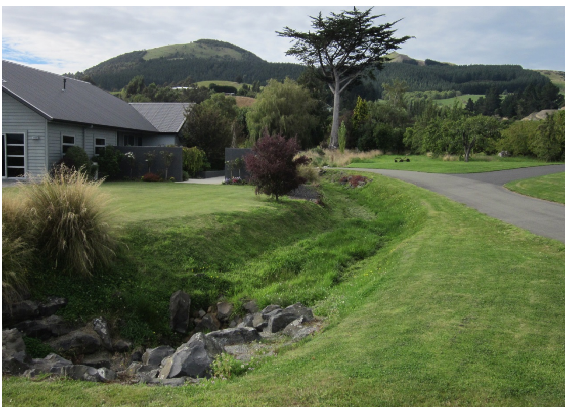
Figure 11 The engineered channel of Jaffray Stream at Orchard Grove, East Taieri. The head of its ~70 hectare catchment extends between Saddle Hill (left) and Jaffray Hill (right). Photo: D.J.A. Barrell, 17 February 2014, GNS Science.
