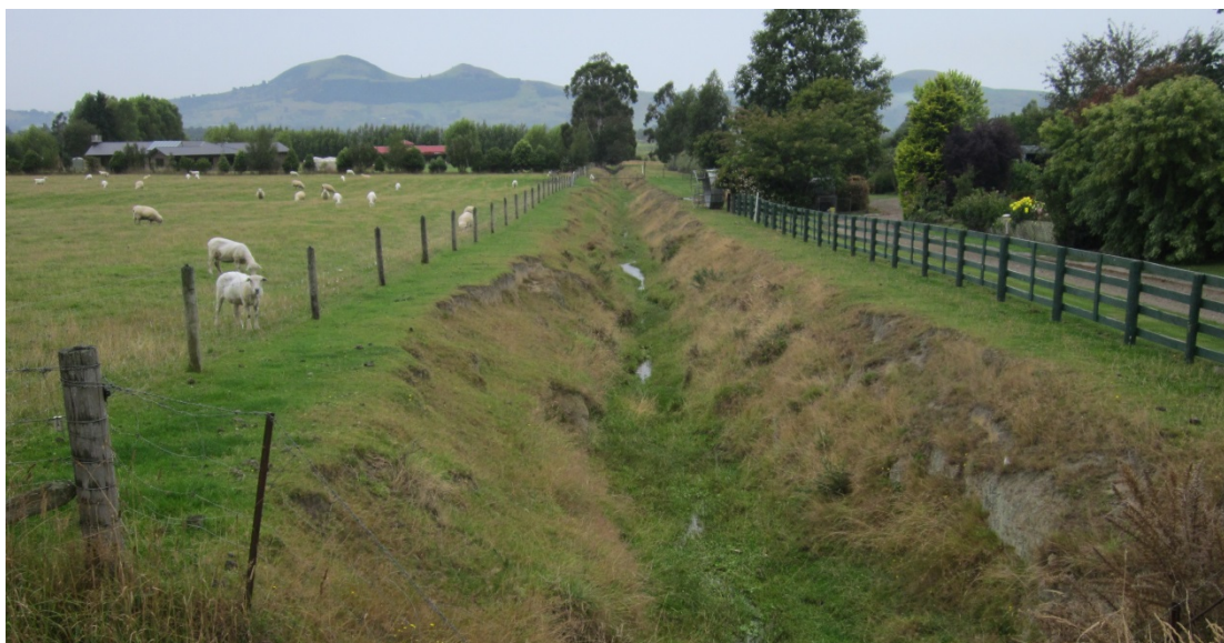
Figure 6 A view southeast from Tirohanga Road, about 0.6 km east of Outram-Mosgiel Road, showing a large artificial channel. There are no deeply inset natural channels on this fan, and doubtless motivated the excavation of this ~3 m deep ditch to capture and convey the runoff from the ~100 hectare hill catchment of this fan. Photo: D.J.A. Barrell, 17 February 2014, GNS Science.
