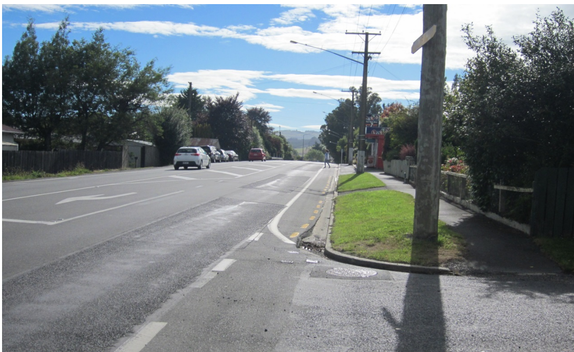
Figure 10 A view northeast along State Highway 1 at East Taieri township, showing the fan of Jaffray Stream. The road rises over the fan axis, and Jaffray Stream is conveyed under the road in a culvert at the point where the road goes out of sight. If the culvert were to become blocked by debris during a major rainstorm, there is potential for flooding and sedimentation on the fan surface. Photo: D.J.A. Barrell, 17 February 2014, GNS Science.
