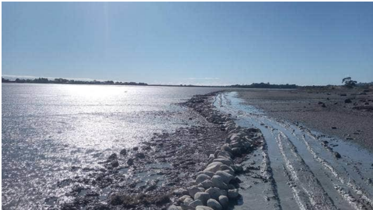
Figure 6. A ‘Chenier sill’ close to the mouth of the Orchard Stream in Stoke, near Nelson. Small boulders increase the height of the estuary bed over time and change the shape of the shoreline to make it more suitable for saltmarsh vegetation to grow. [Photograph supplied by Nelson City Council].
