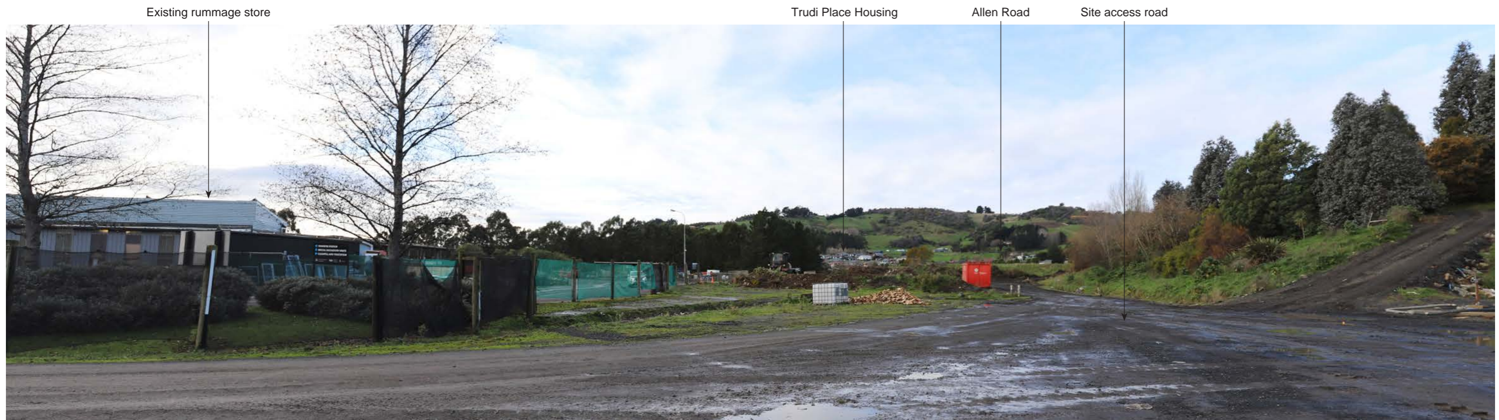
Site Appraisal Photograph B: Photograph taken from the access road of the Site, looking in a southeasterly direction across the proposed locations for the Materials Recovery Facility and Bulk Waste Transfer Buildings, and worker facilities.
