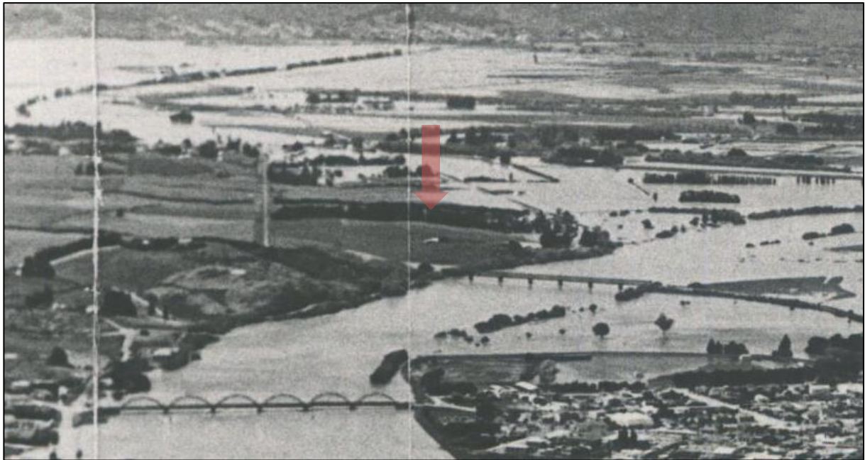
Figure 5-7. Detail of photograph 1957 photograph, with the cottage indicated (O.D.T. Collection, 1957).
