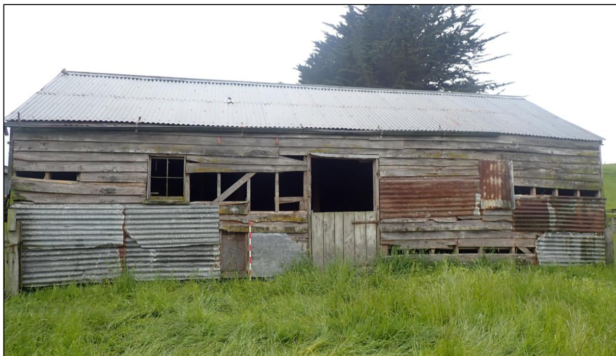
Figure 7-12. East elevation of the stable, now shearing shed.
