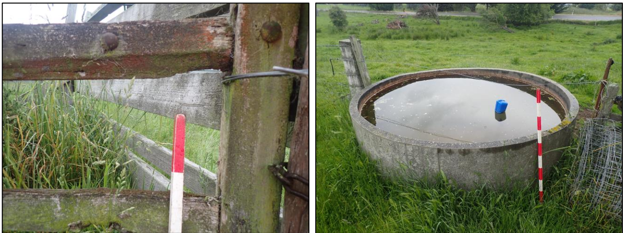
Figure 7-9. Left: Coach bolts in fence with modern wire wrapping. Right: concrete trough at end of fence.
