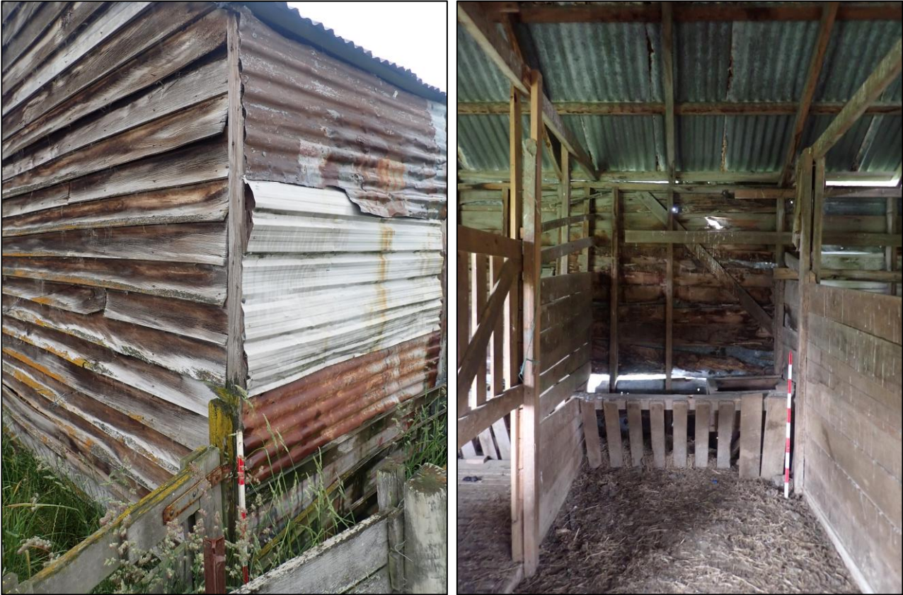
Figure 7-13. Left: north corner of stable, showing meeting of two phases of cladding. Right: stall within stable, showing the original partitions and modern additions.
