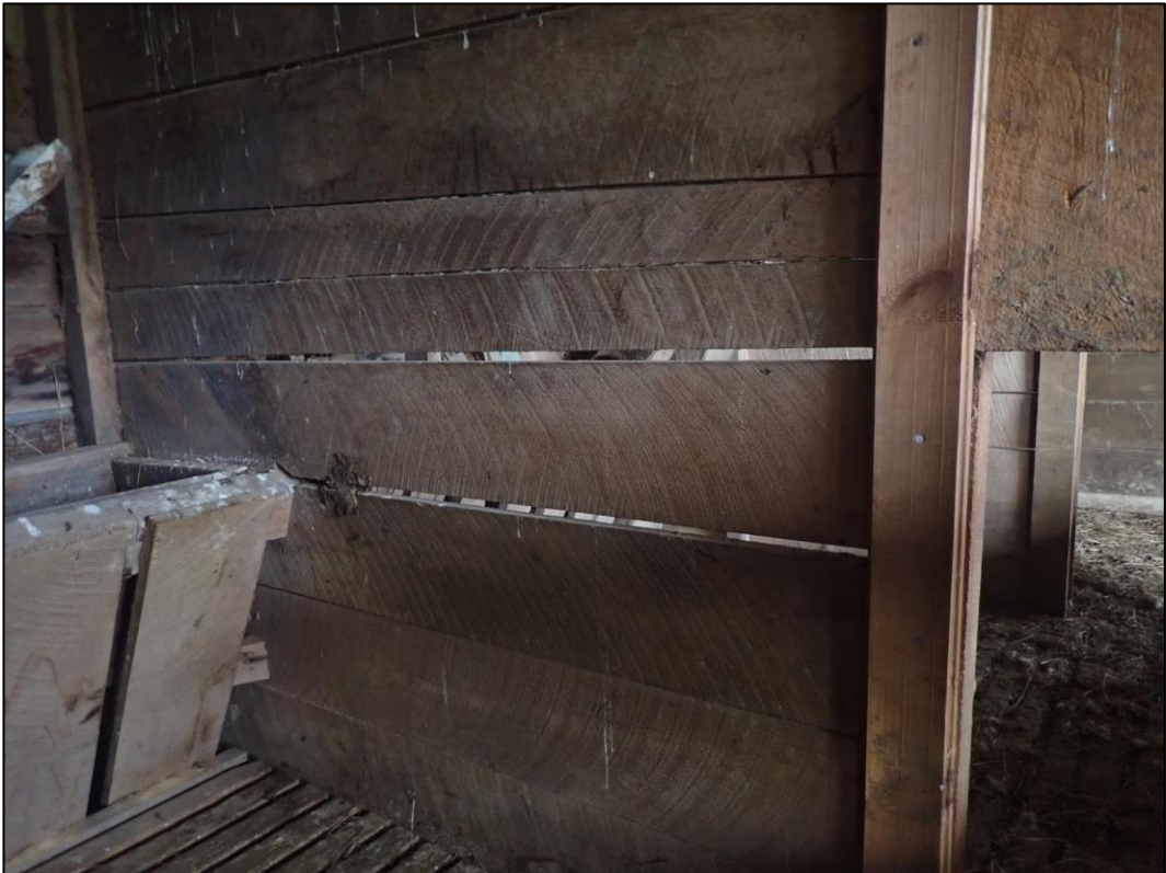
Figure 7-14. Pit sawn timbers used for the partitions between stalls.
