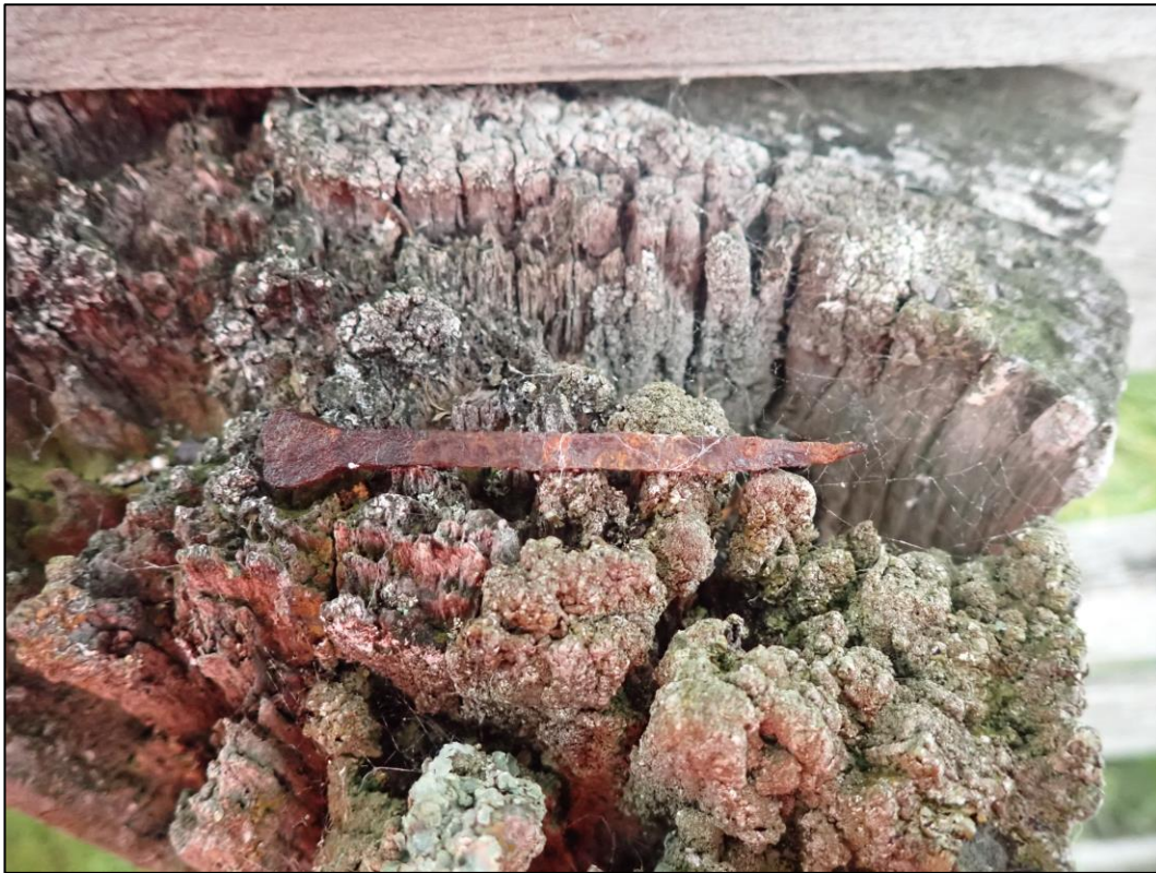
Figure 7-10. Wrought nail found on fence post, matching others still in situ.
