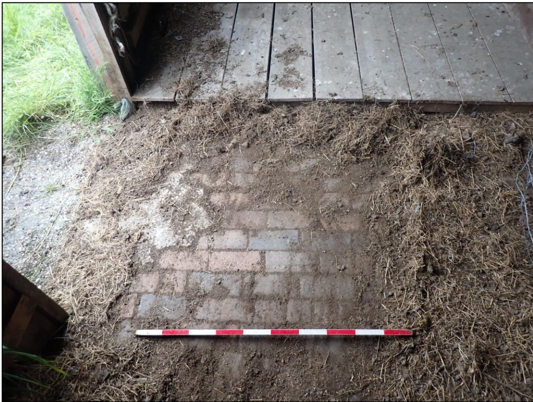
Figure 7-16. Brick floor with modern timber added over.
