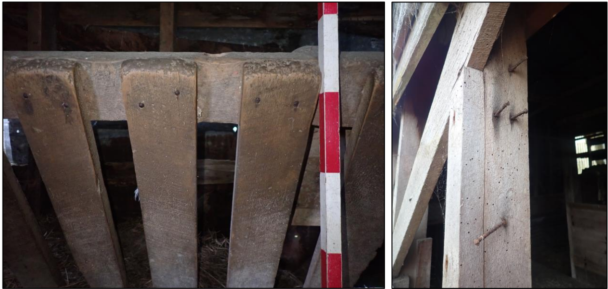
Figure 7-15. Left: Pit sawn timbers and rose-head nails on feed troughs. Right: rose-head nails used in wall framing.
